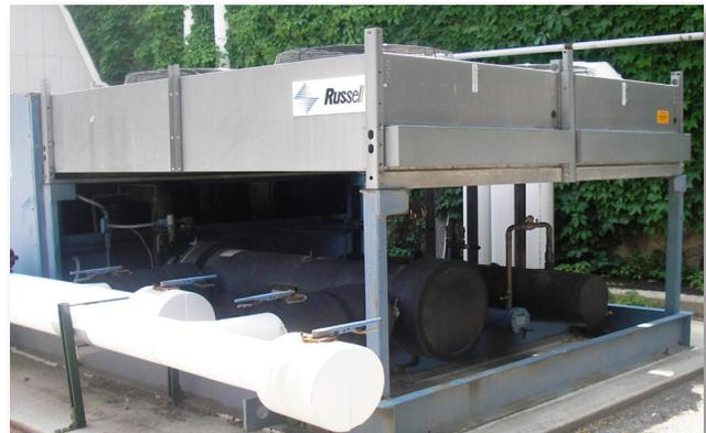
Chiller used to keep temperatures between 40-45 degrees
